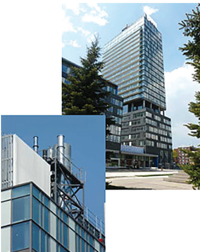
Figs 15 & 16. Regent Park’s 22 – story building with district heating plant (inset). Courtesy of Doug Pollard
