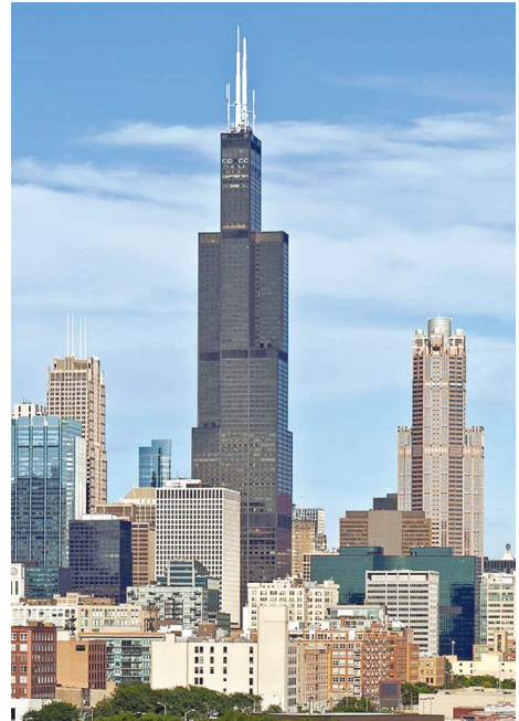
Fig. 10. The Willis Tower, Chicago (source: [20])
