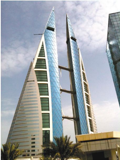
Fig. 21. The Bahrain WTC building has three 29-metre high wind turbines. Image courtesy of Wikipedia (By Fred Hsu [30, 31])
