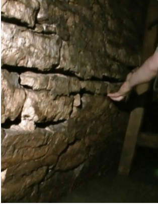
Fig. 5. View of "Fryderyk" adit in the area of point 25 on Fig. 4 [10]
