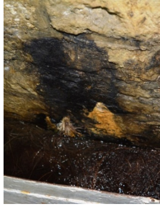
Fig. 6. View of "Fryderyk" adit in the area of point 20 on Fig. 4 [10]
