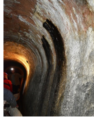
Fig. 7. View of "Fryderyk" adit in the area of point 9 on Fig. 4 [10]
