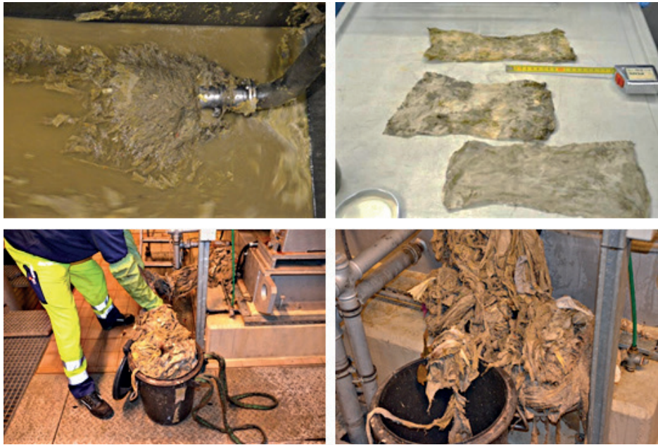
Fig. 4. Impressions of wet wipes in the Berlin sewer system [pictures from TUB-FSD and BWB]
