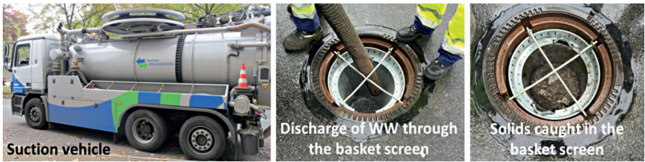
Fig. 6. From left to right: Suction vehicle, wastewater being discharged into the basket screen, basket screen retaining the solid
