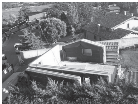
Fig. 5. The construction of a “Haus Larix” house (2013) [9]
