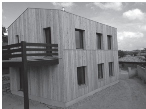
Fig. 4. Wooden building envelope [9]
