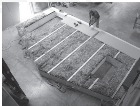
Fig. 6. Prefabricated elements based on wood and straw [9]
