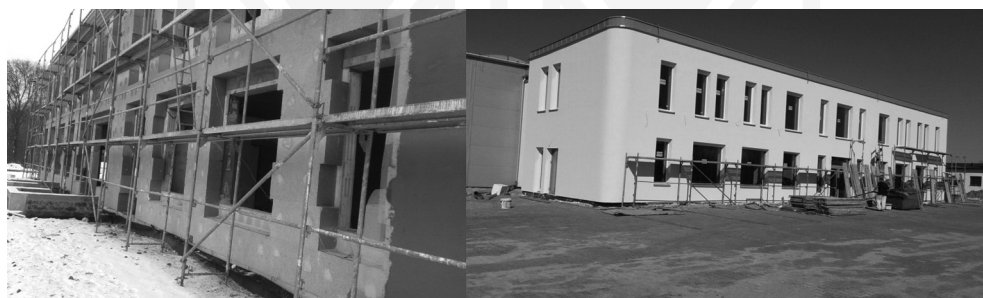
Fig. 1. Office building under construction as part of the EU project (PCBP)
