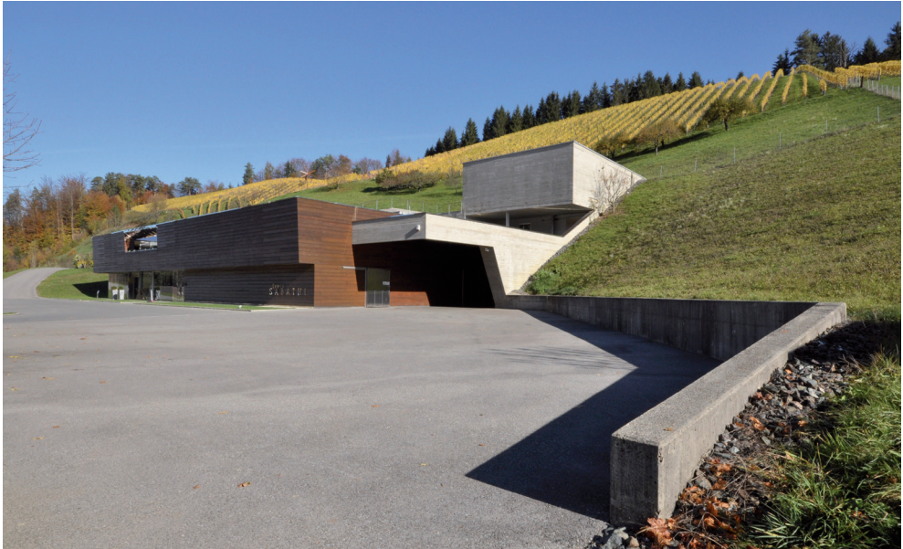
III. 11. Erwin Sabathi's wine manufacturing facility, located in Pössnitz – as of 2013 (photo by K. Zawada-Pęgiel)
