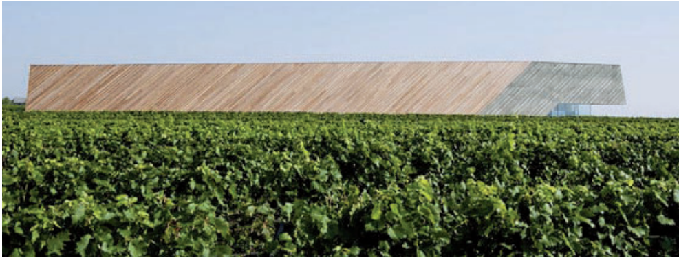
III. 7. The external façade of Claus Preisinger’s wine manufacturing plant, site near Gols (photo by Herth Hurnaus; source: http://www.dailytonic.com/claus-preisinger-vineyard-by-propeller-z-at , online: 19.02.2015)
