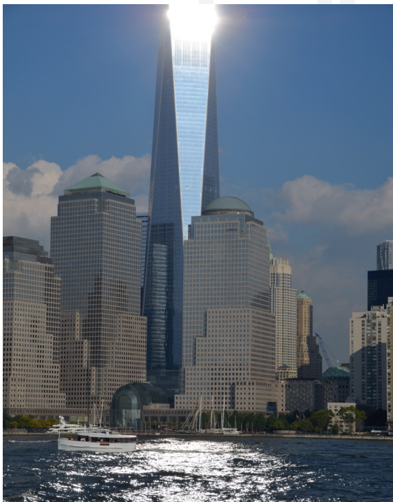
III. 2. Freedom Tower (ground zero) the tallest Tower of Manhattan (105 floors, 1776 ft – its height is the symbol of the date of Declaration of Independence). One of four, which are part of a new development created in place of WTC. Authorship: Daniel Libeskind, David Childs, Skidmore, Owings & Merrill (photo by author, 2013)
