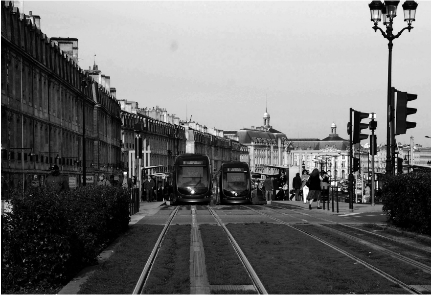
Ill. 4. Green track, and the ‘third’ power line, Quai Richelieu in Bordeaux. Photo by the author
