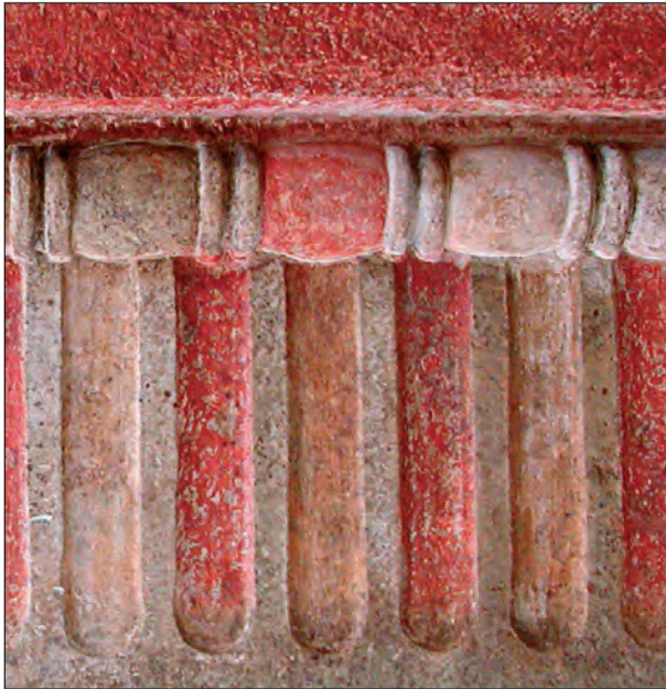
Fig. 6. Old Nisa, Red Building: particular of the stone slabs socle of the façade
