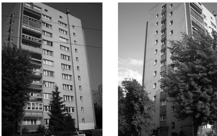
Fig. 1. North and East elevations of analyzed building
