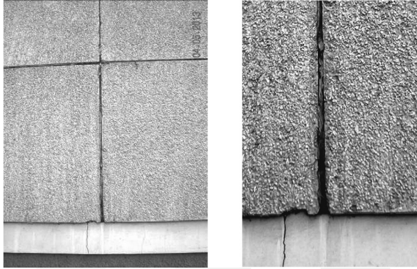
Fig. 2. Panel connection joint – external view
