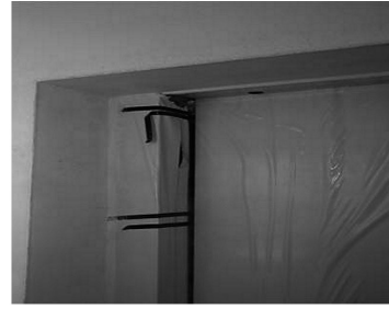
Fig. 4. Preparation of lift shaft
