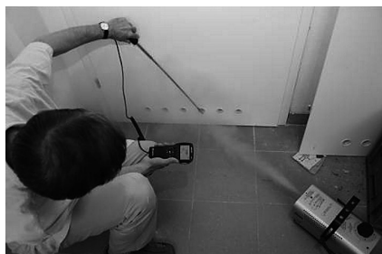
Fig. 5. Detection of leakages with fog generator and anemometer
