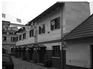
Fig. 1b. Building B
