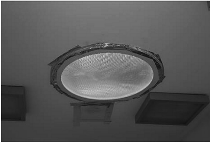
Fig. 3. Preparation of lighting fixtures
