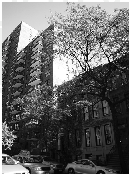
III. 24. A new apartment block in 92nd Street, in Manhattan. Next to it traditional New York tenements after restoration (photo by D. Kuśnierz-Krupa, 2010)
