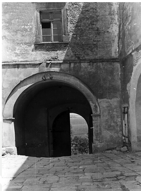
III. 12. Courtyard of the castle in Olesko at the beginning of the 20th century (Archive of the Department HAUiSzP WA PK, s.v.)
