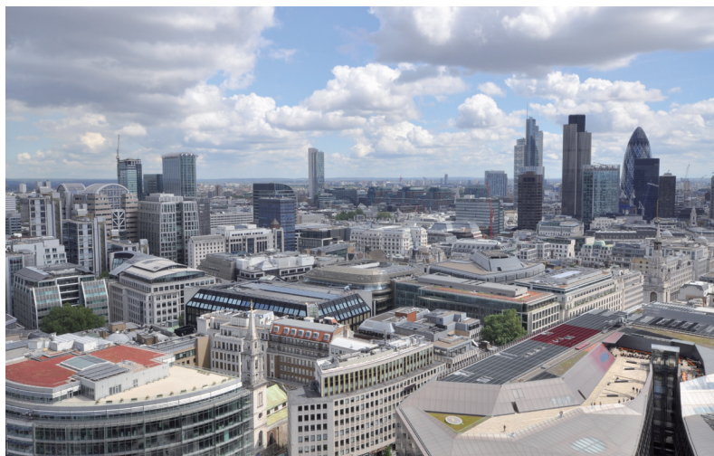
III. 3. City of London from the top of St Paul's. The view is showing low and high office buildings (photo by Katarzyna Zawada-Pęgiel, June 2012)
