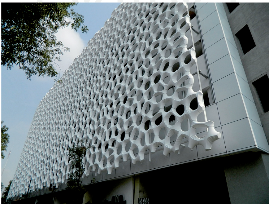
III. 10. A Prosolv de-polluting facade is installed at Hospital Manuel Gea Gonzales in Tlalpan (Image: Prosolv)
