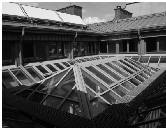
III. 3. Glazed atrium at the level of the second floor
