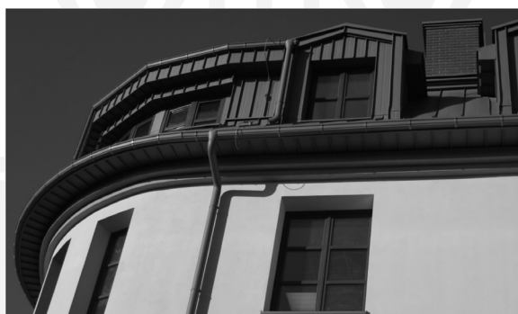
III. 7. Fragment of a part of the roof dormer covered with plate
