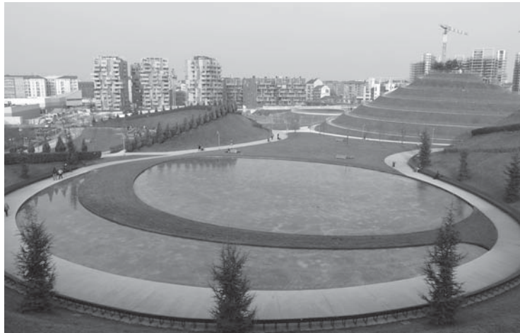
Il. 8. A view of the former Maserati Industries area at the Portello Park (photo: LMF Fabris, 2015)
