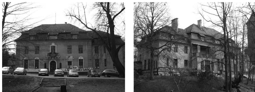
Fig. 1, 2. The front and back elevations of Villa Casablanca, before the renovation in 2006
