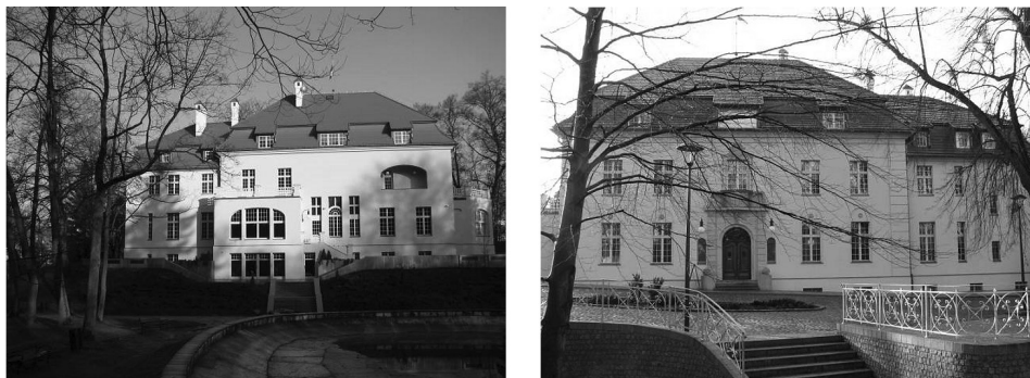
Fig. 27, 28. The front and southern Casablanca elevations after the renovation, 2014
