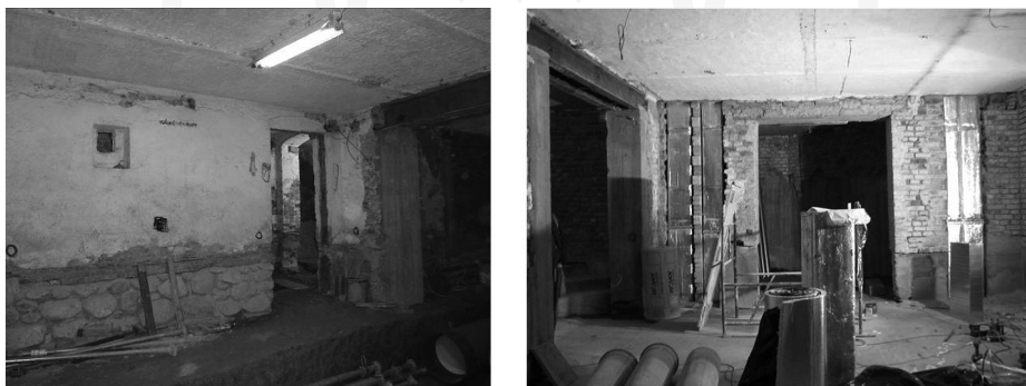
Fig. 21, 22. The works of deepening the cellar, 2011
