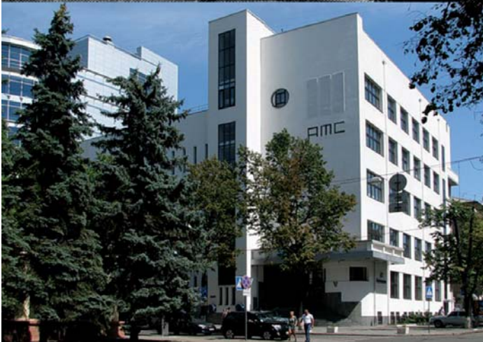
il. 8. Building of ATS. Pavel Frolov. 1930–1932
