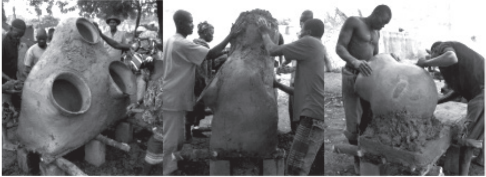
Ill. 18. Women's Association Centre in Gando. Burkina Faso. Casting of clay vessels used to store food products in the wall (source: [7])
