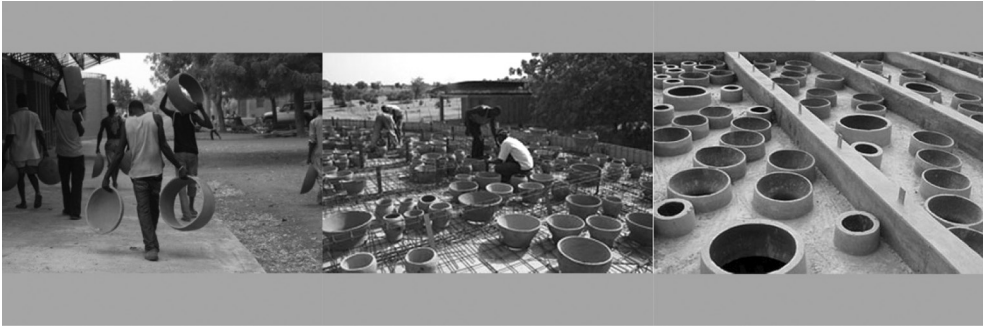
Ill. 16. Library in Gando. Burkina Faso. From left: Arranging trimmed ceramic vessels in the reinforcement of the floor slab and the finished floor (source: [2])
