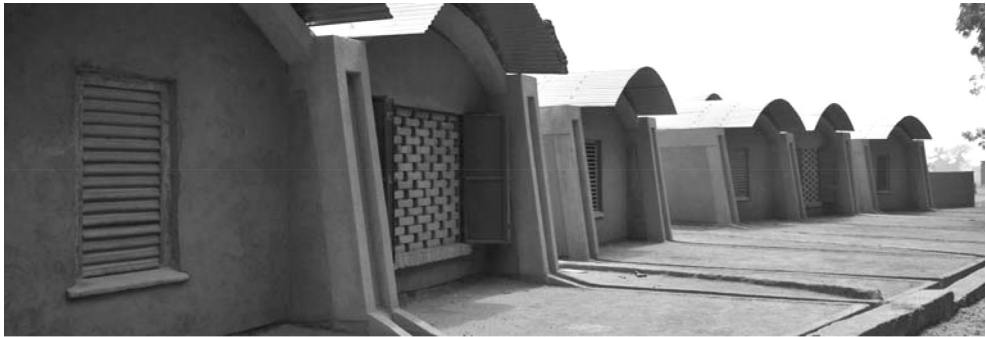
Ill. 11. Teachers housing in Gando, Burkina Faso. Openwork, ventilated front elevation (source: [8])
