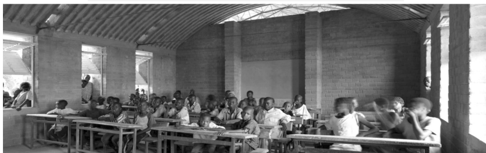
III. 3. School in Gando, Burkina Faso. Classroom with a prominent barrel vault, which contains ventilating holes (source: [1])
