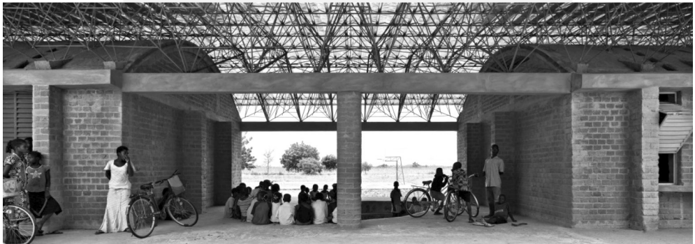
III. 5. School in Gando, Burkina Faso. The amphitheater recess, covered with steel roof truss – a playground and a meeting place for children (source: [1])
