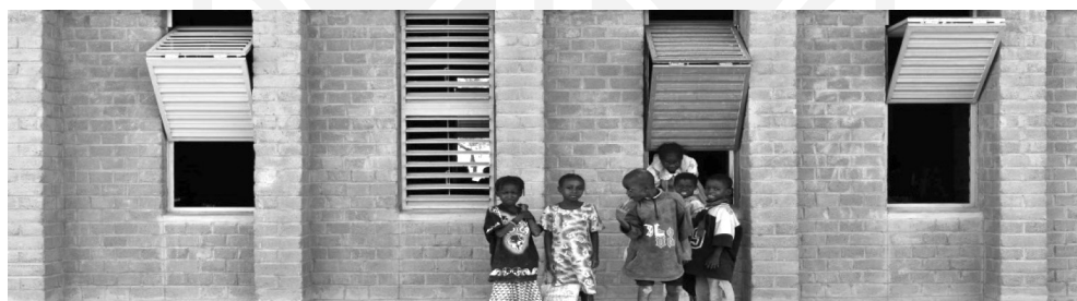
III. 2. School in Gando, Burkina Faso. Colourful, openwork shutters (source: [1])
