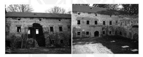
Fig. 2. View of the administration wing and repairs which have been made using ceramic brick. Left side is a view on the day of February 2nd, 2013 to the right as at September 28th, 2013
