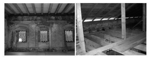
Fig. 3. Wooden beam-framed floors restored in the north wing of the palace
