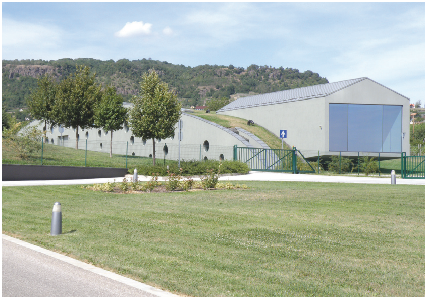
Fig. 4. View of Champagne maturing facility, “Greater Somló” wine district (photo by M. Simon, 2017)
