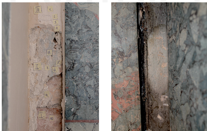
Ill. 4. Wrocław, 6 Rynek, traces of bluish paint from the first chronological phase (photo by Wiesław Piechówka)
