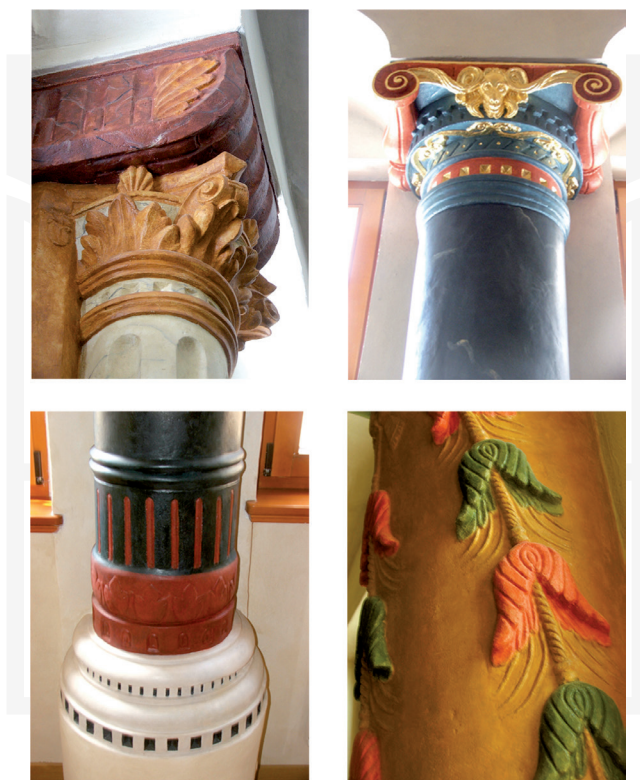
Ill. 2. Wrocław, 4 Kurzy Targ Street, the Renaissance colour schemes on internal columns after conservation-details (photo by the author)
