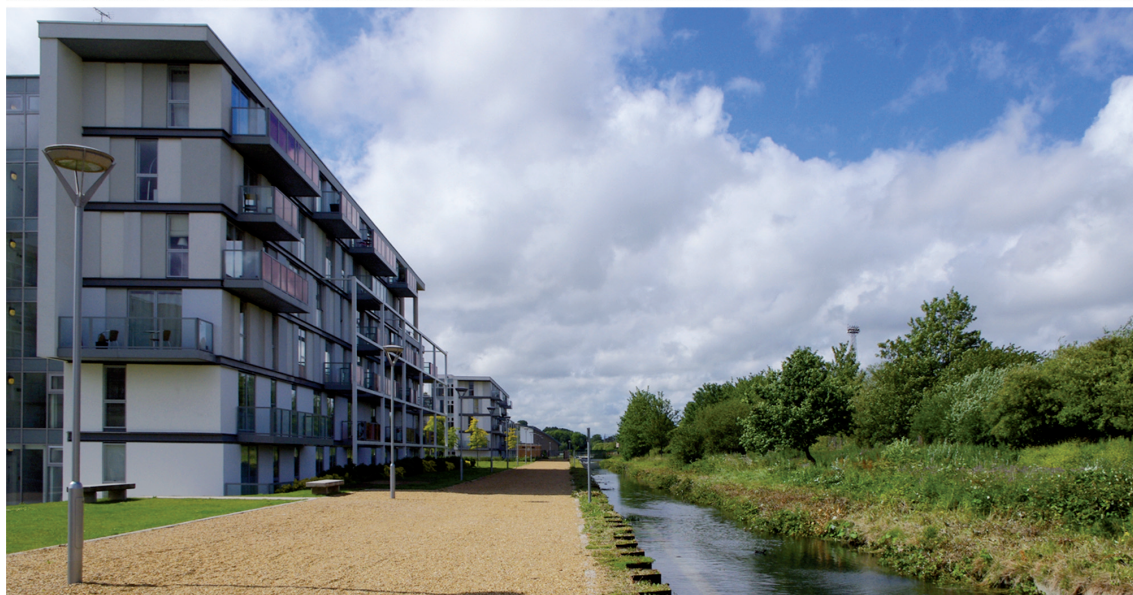
III. 4. New River Village housing estate – linear park along the river (photo by E. Kusinska)
