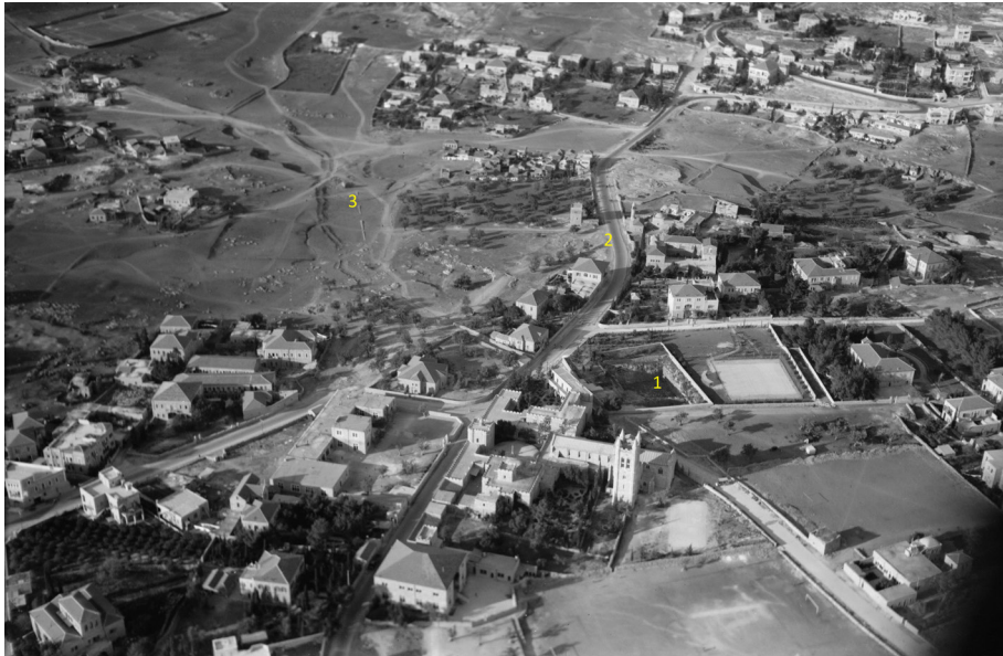
Fig. 2. Oblique aerial photograph of the area north of the Old City of Jerusalem taken on Nov. 10, 1933: Note the Tombs of the Kings (1) adjacent to Nablus road (2) and earlier road to NW (3) marked also in Fig. 1 (Photo by unknown photographer; American Colony (Jerusalem) Photo Dept., Matson Photograph Collection; Library of Congress, Washington, D.C. LC-DIG-matpc-22157)
