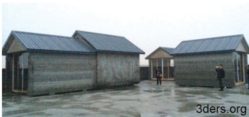
Fig. 2. Examples of buildings printed using 3D printing technology – carried out in Shanghai by Shanghai WinSun Decoration Design Engineering Co. [10]
