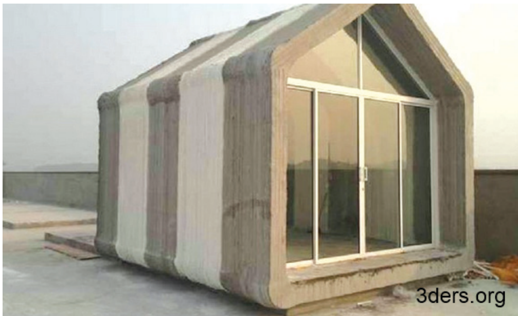
Fig. 3. Example of a building printed using 3D printing technology – by Shanghai WinSun Decoration Design Engineering Co., Shanghai, China [10]
