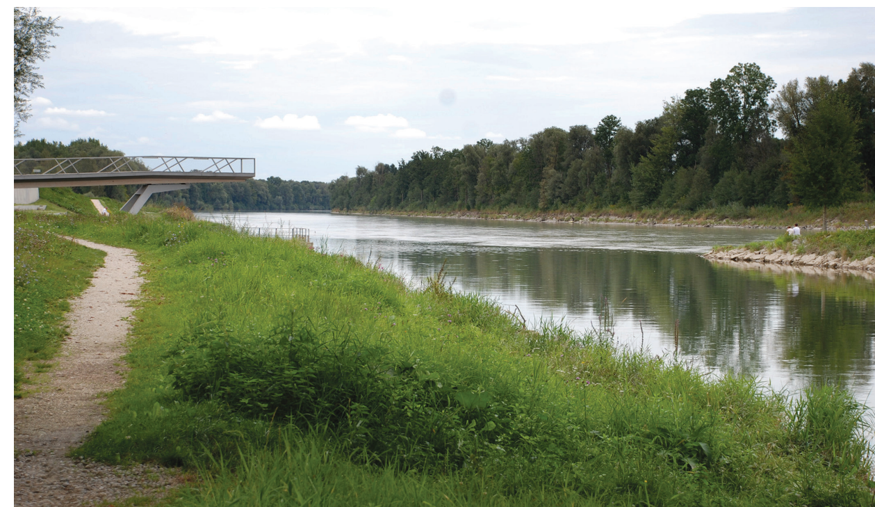
III. 5. Flood protection improvement, biodiversity increase, spaces for recreation on the riverbank. Rosenheim, river Inn. Credit: P. Kowalski, 2012
