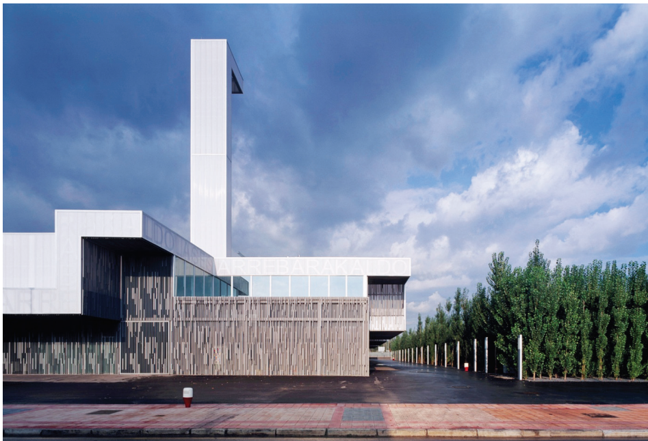
Fig. 8. Lasarre Barakaldo Stadium, Barakaldo, facade with semi-transparent, backlit panels and steel grates, phot. by Roland Halbe (source: [43])
